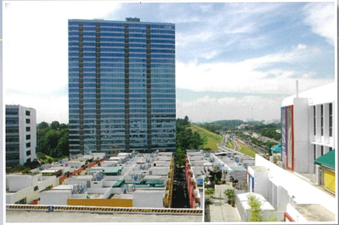
WCEGA Building & The Splendour
