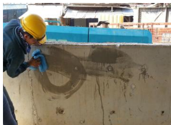
Damp the substrate with water
