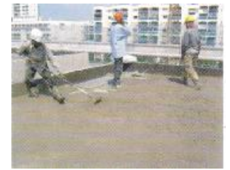
Casting of topping concrete after expansion joints are laid
