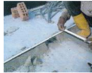
Marking out using strings
