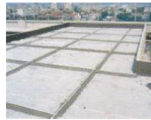
Expansion joints laid in grids with mortar
