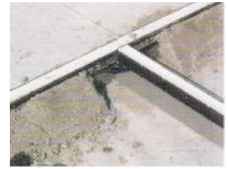
Positioning and securing of expansion joints on both sides with mortar
