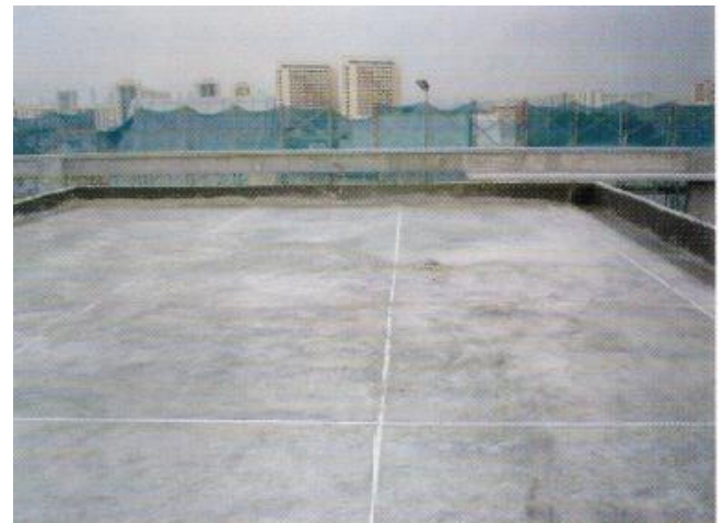
Final finished product. White tape on top of the PVC capping may be removed.
