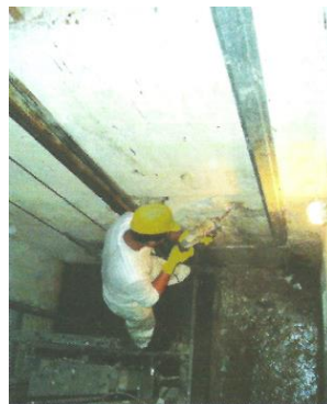
Drilling hole into the substrate that has water leakage
