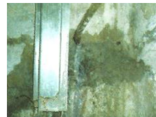
CL-PUJet is pumping into the hole via packer
