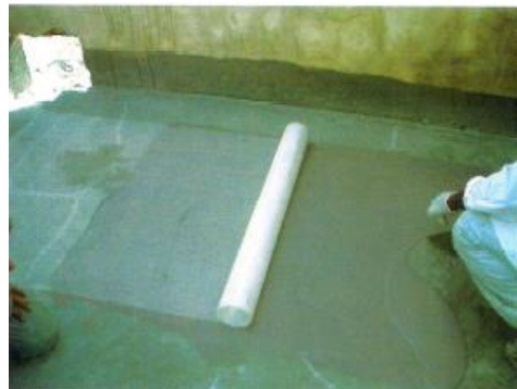
Lay CL-Fabric into first coat while it is still wet
