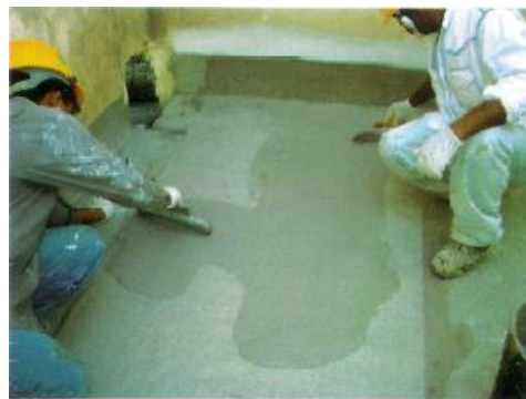
Apply second coat of waterproofing on wet-on-wet basis and sandwich CL-Fabric in between
